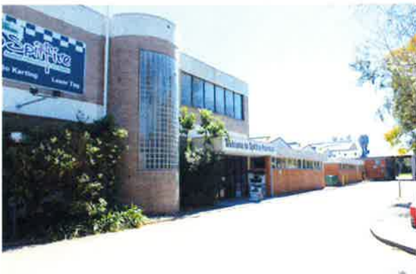
Figure 2: Existing buildings on site.
